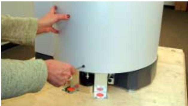
Unscrew the screw in the lower part of the front panel, using the flat screwdriver.
